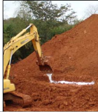
Application of caustic soda to soil in the AH Process
