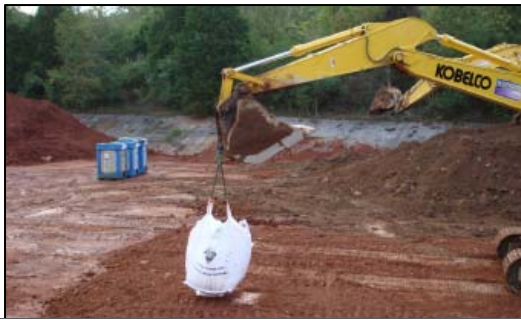
Example of how chemicals are introduced to the soil
