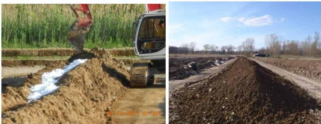
Figure 3. Application of anhydrous pellets of NaOH for alkaline hydrolysis of soil using a windrow treatment configuration at the former Plum Brook Ordnance Works (PBOW)
